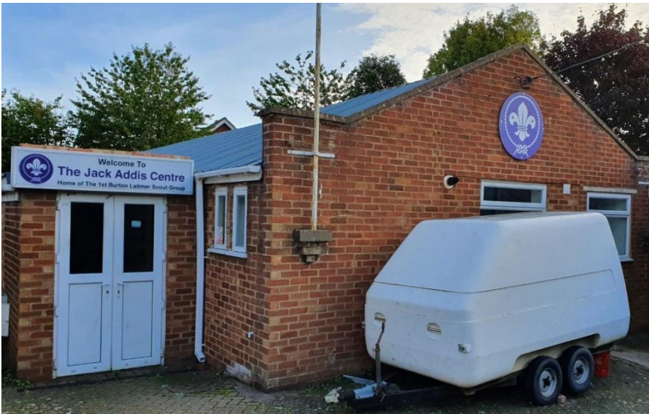
The Jack Addis Centre, Burton Latimer
