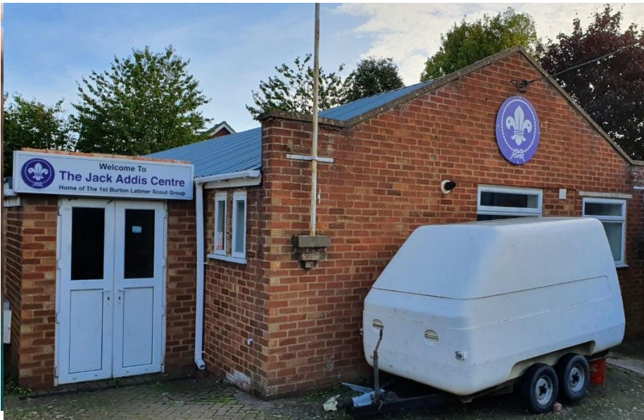
The Jack Addis Centre, Burton Latimer
